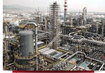
IRAK HEAVY FUEL OIL (MCC ADP Panoları)
